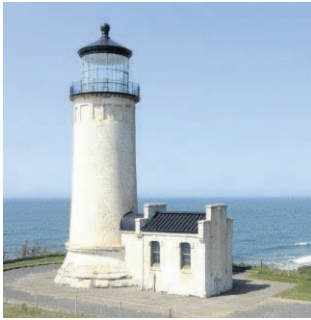
SUBMITTED PHOTO BY STEPHEN WOOD/ CAPE DISAPPOINTMENT STATE PARK The North Head Lighthouse is undergoing restoration. Its red roof was painted black last year.
