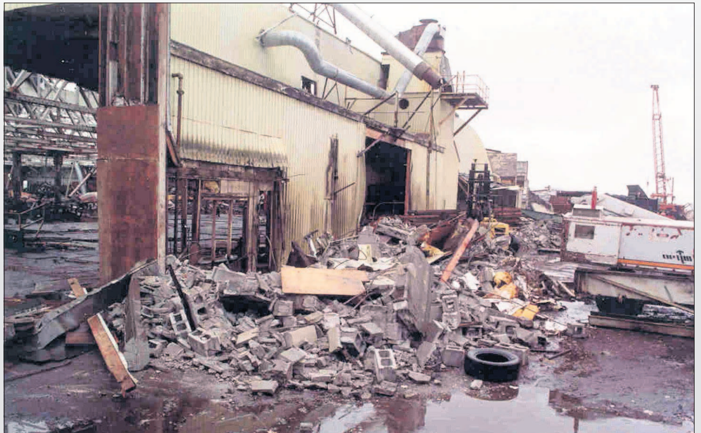
One of the Astoria Plywood Mill’s buildings.
