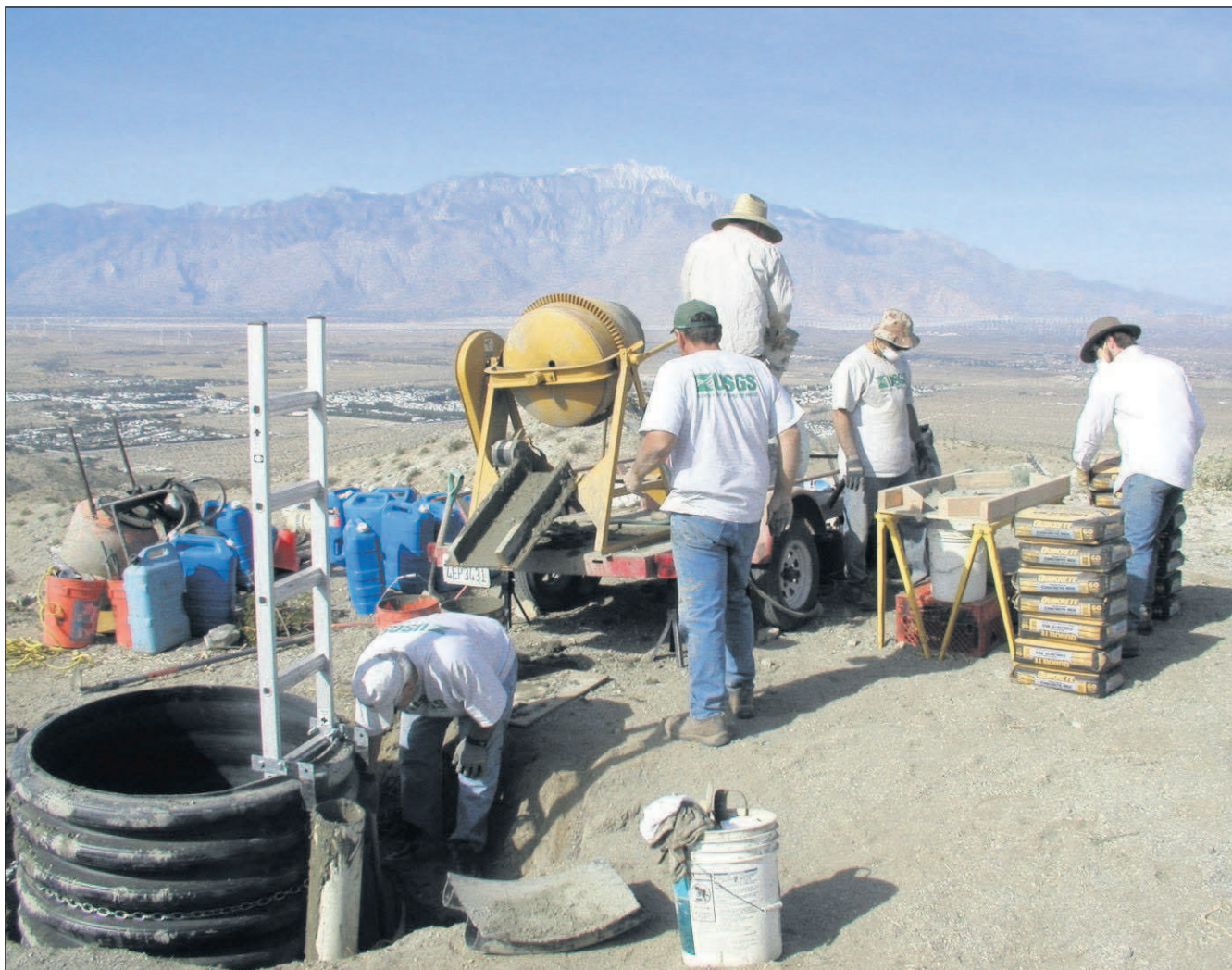
Crews work to install the earthquake sensing equipment in California.
