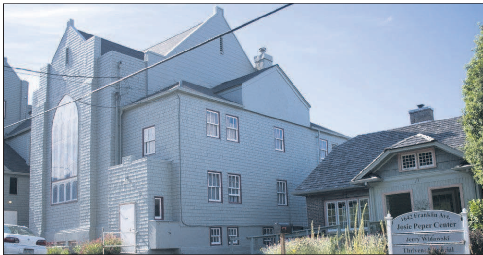
The Daily Astorian Clatsop Community College has received an offer on the Performing Arts Center, left, and Josie Peper Building.
