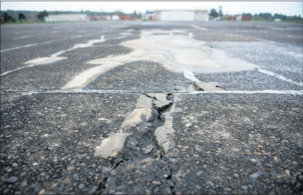
Photos by Joshua Bessex/The Daily Astorian The Port of Astoria is facing cracks, depressions and uneven concrete slabs at the Astoria Regional Airport, which some have said might be caused by nearby wetlands.
