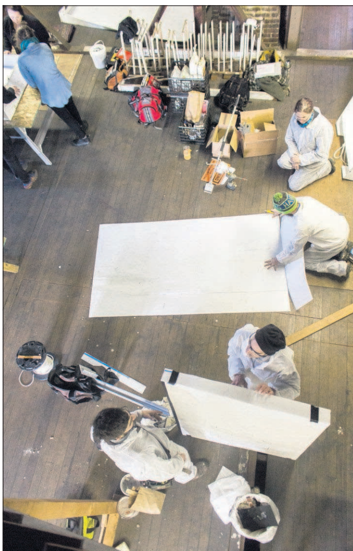
Students in Clatsop Community College's historic preservation and restoration program took over the attic of the Flavel House Museum over the weekend. They restored the sash windows in the attic of the 131-year-old mansion.
