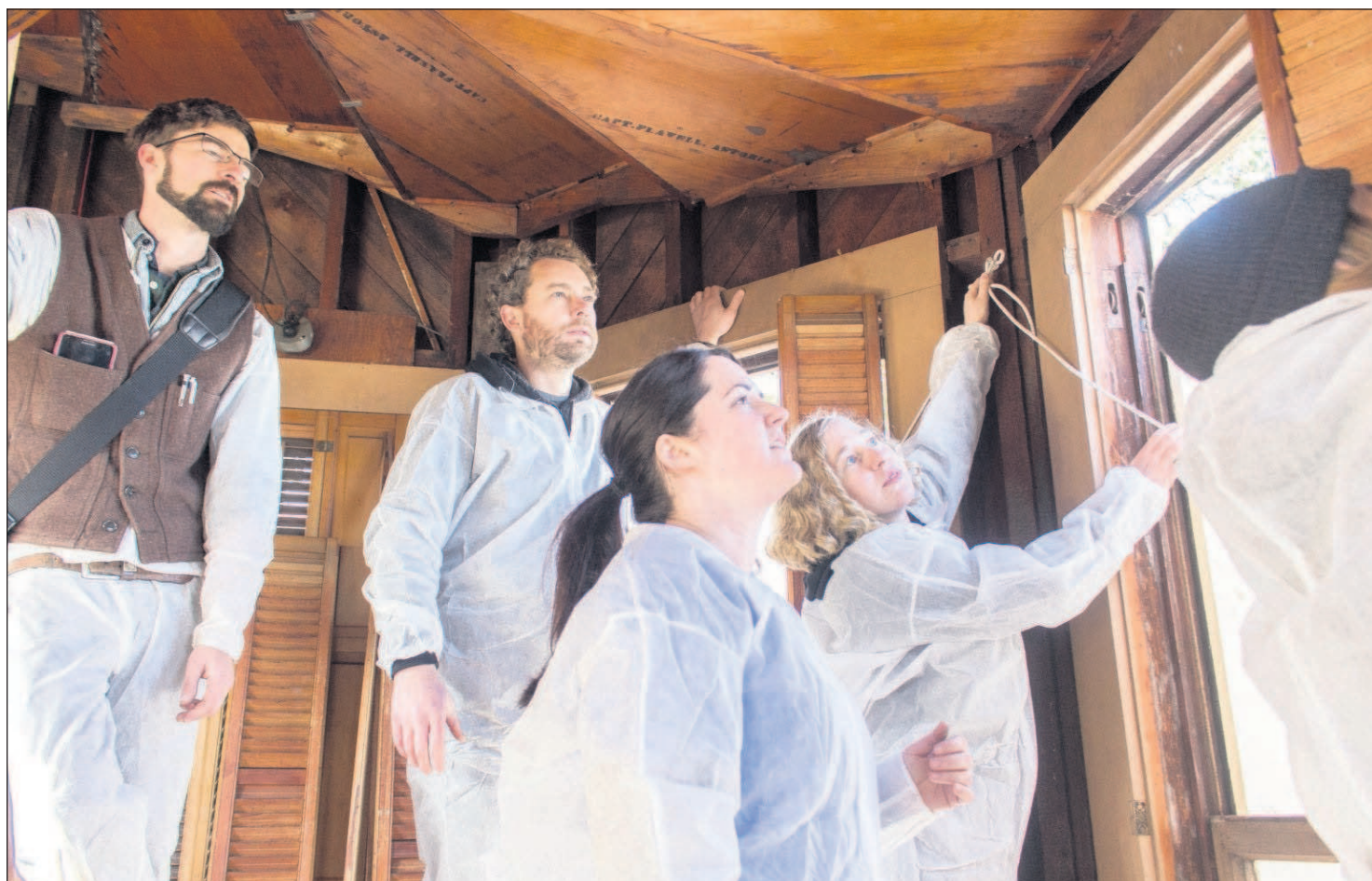
From left, instructor Chris Gustafson, a graduate of Clatsop Community College's historic preservation and restoration program and a professional window restorer, teaches students Jay Dickason, Chelsea Billings, Hannah Phelps-Goodman and Alisyn Smith how to remove the sash windows in the 131-year-old Flavel House Museum and contain their work area using corrugated plastic sheeting.
