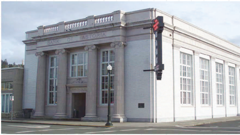
RICKENBACH CONSTRUCTION PROJECT | 2007
