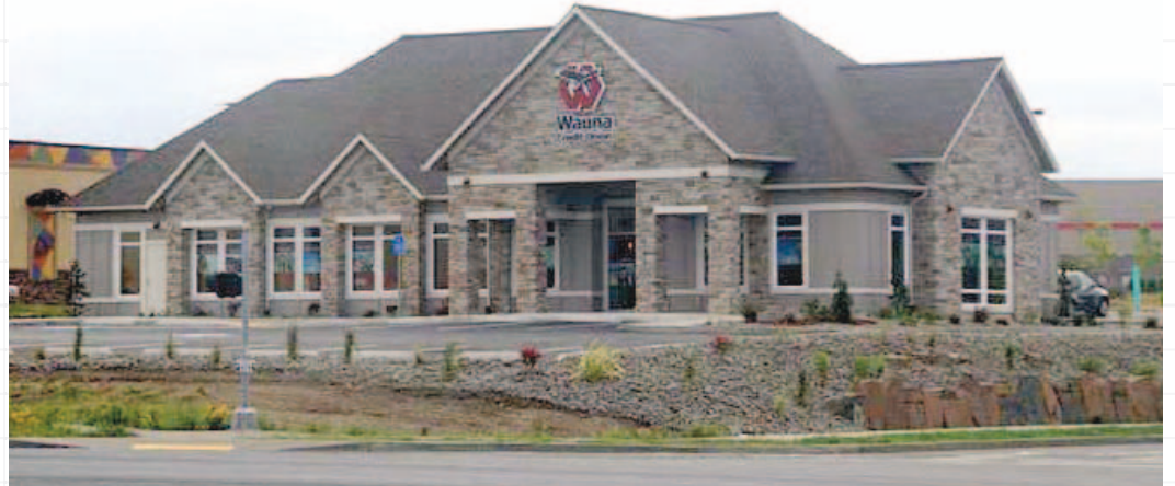
RICKENBACH CONSTRUCTION PROJECT | 2013
