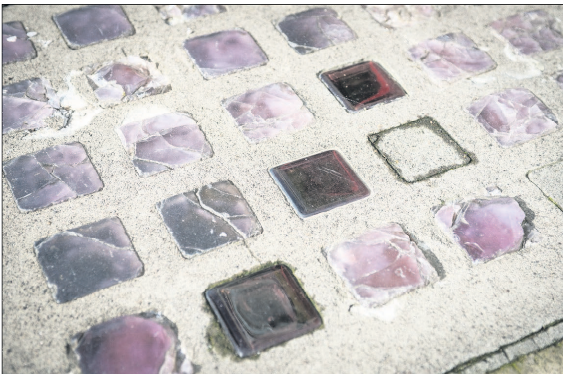
New glass tiles fill gaps in the sidewalk near the Carruthers Building. Joshua Bessex/The Daily Astorian
