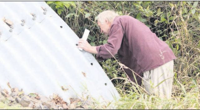
Katherine Lacaze/EO Media Group A workshop participant looks through the Hawley Creek arch, a structure that replaced a fish passage barrier culvert during a project in 2007.
