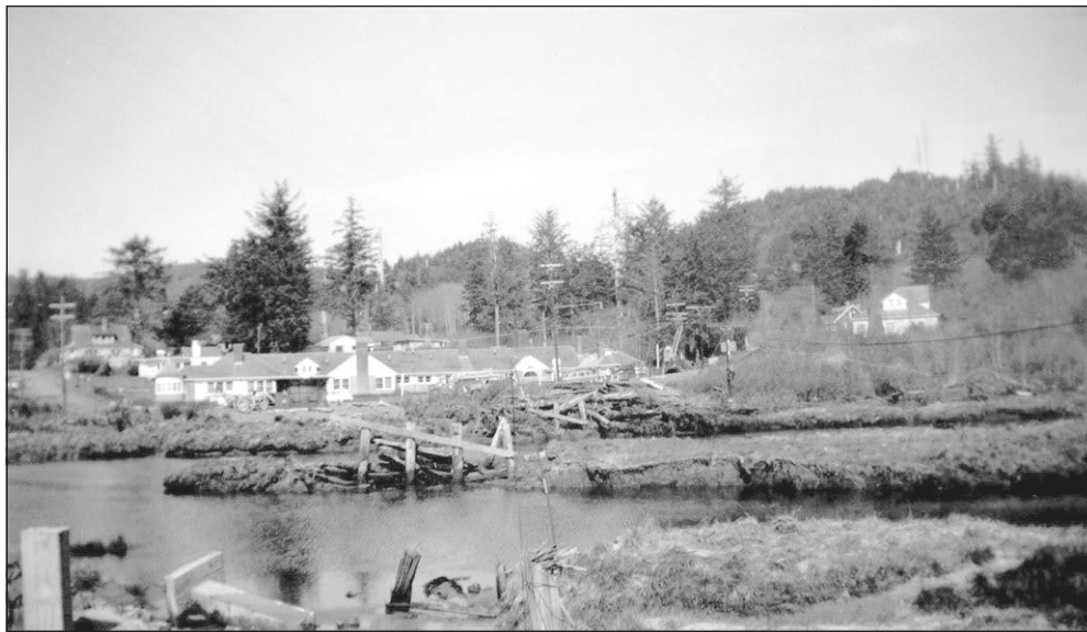
Submitted Photo/Cannon Beach History Center A bridge went out during the 1964 tsunami. Officials fear an earthquake or tsunami could wreak havoc with the city's current system.
