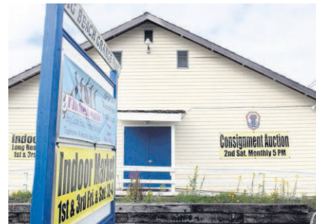
Thanks to the work of dedicated members, the Long Beach Grange hall has been restored with new windows, LED lighting, a new roof and a handicapped-accessible front entrance. Now, the sturdy building serves as a thriving community meeting place.
