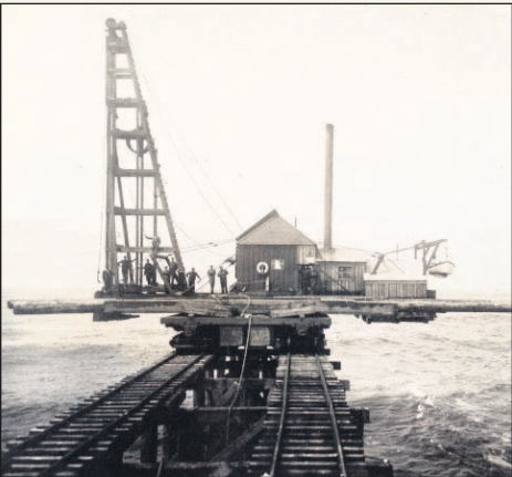
Courtesy of the Clatsop County Historical Society A large pile driver trundles along, extending the railroad trestles that will eventually be closed in with piles of rocks and become South Jetty.
