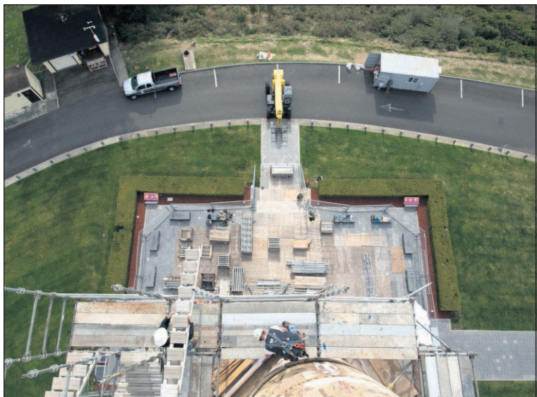
Crews remove stairs and scaffolding from around the Astoria Column Tuesday.
