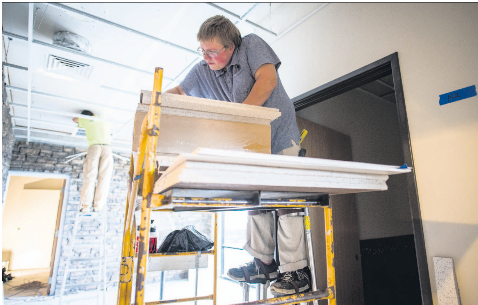
Andrew Midkiff cuts acoustical ceiling tile to install in the new Oregon State Police Astoria Area Command Center.
