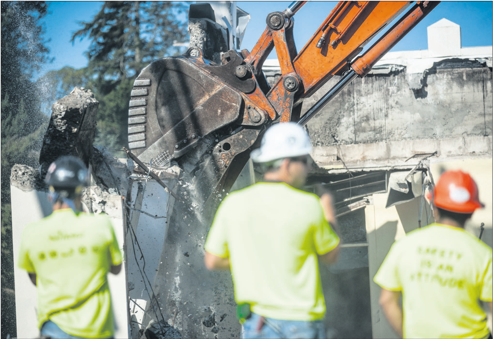
Crews with P&C Construction watch as an excavator tears down the walls of Patriot Hall Tuesday. Patriot Hall is the third phase of Clatsop Community College's Jerome Campus Redevelopment Project, and will become a modern gym and academic hall by fall term 2016.
