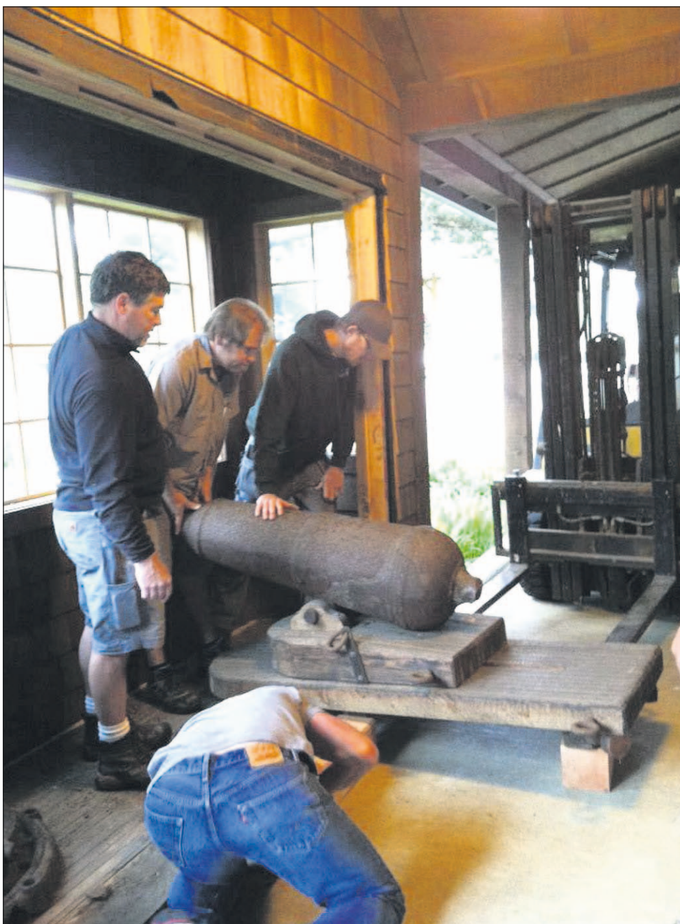
A crew from Coaster Construction works to get the USS Shark cannon out of the Cannon Beach History Center and Museum.
