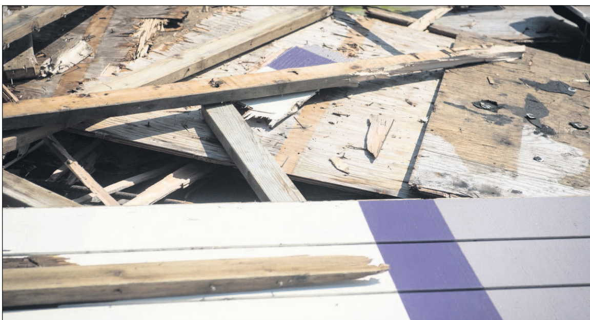
Siding from the grandstands rests in a pile.
