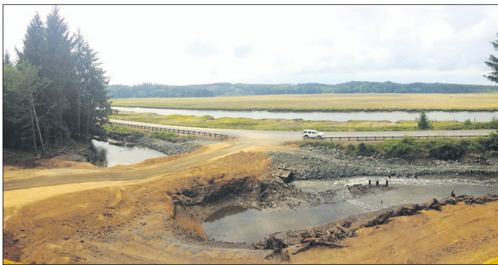
Madeline Kalbach/Submitted Photo A newly installed box-style culvert provides tidal-level access to extensive acreage south of U.S. Highway 101 near Long Beach, Wash.
