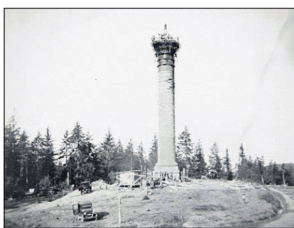
Courtesy Clatsop County Historical Society The Astoria Column during construction in 1925.
