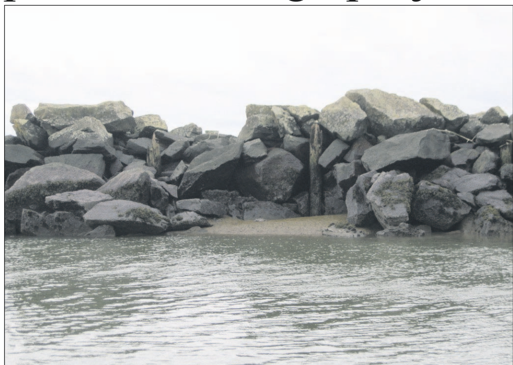
Gail Sandana/Submitted Photo Massive jetty stones, some weighing up to 7 tons, armor Trestle Bay. In 1995 the U.S. Army Corps of Engineers removed a 500-foot section of the 100-year old jetty to allow salmon and steelhead greater access to quieter, tidally influenced water. The Corps will remove another 900 feet in various sections this fall. The Trestle Bay restoration was developed after the success of the initial notch.
