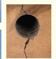
Core samples were taken to get a better understanding of the condition of the concrete. Vertical cracks were visible within a decade after the column was built in 1926.
