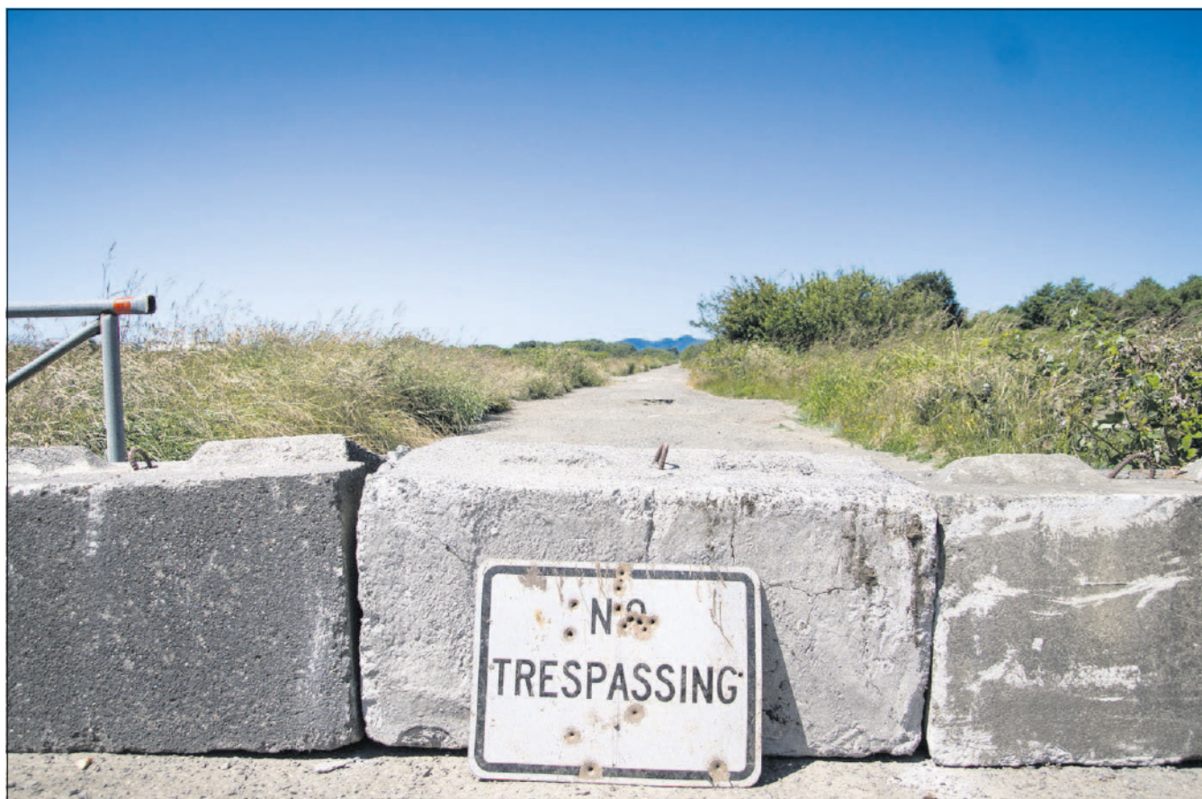
Concrete blocks block the road at the damaged gate along Northeast King Avenue.
