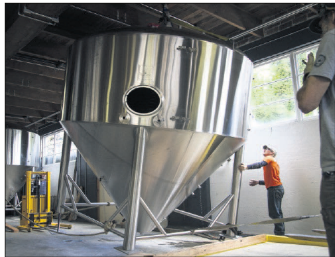
Photos by JOSHUA BESSEX — The Daily Astorian ABOVE: Crews from Fort George Brewery use a crane to unload a fermenting tank from a trailer in the Fort George Brewery courtyard Friday. RIGHT: Michal Frankowicz, with Fort George Brewing, helps steady the fermenting tank as it is lowered into position. In order to pick up the tank, a cable was run through a hole in the ceiling of the brewery and attached to the top of the tank.
