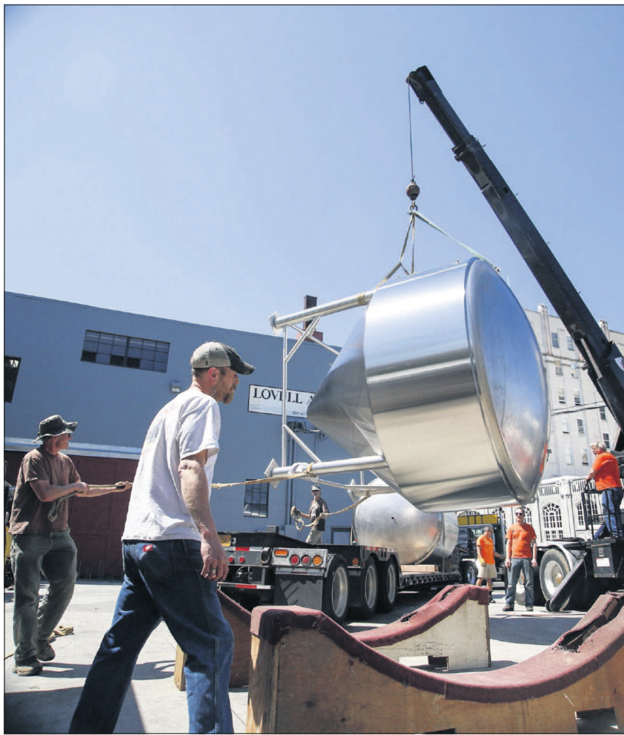
Photos by JOSHUA BESSEX — The Daily Astorian ABOVE: Crews from Fort George Brewery use a crane to unload a fermenting tank from a trailer in the Fort George Brewery courtyard Friday. RIGHT: Michal Frankowicz, with Fort George Brewing, helps steady the fermenting tank as it is lowered into position. In order to pick up the tank, a cable was run through a hole in the ceiling of the brewery and attached to the top of the tank.
