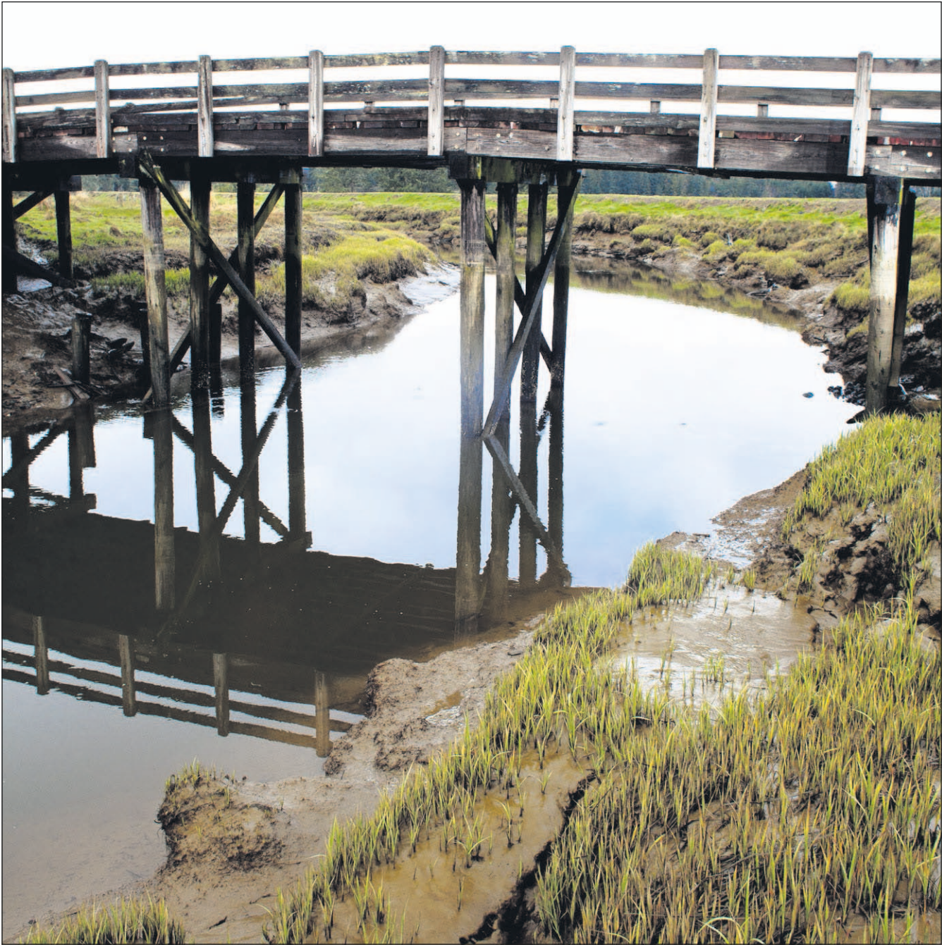
South Nemah River Bridge, located on Lynn Point Road, built in 1959, rated 50. In theory, anything below an 80 qualifies for repairs, and anything below a 40 “bears some careful watching.”
