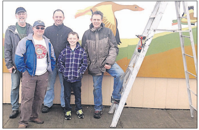
Submitted photo Ilwaco, Wash., Councilman David Jensen, Oddfellow building owner Jeff Cutting, Bruce Peterson, Dustin Mead and Jeff's son Griffin all chipped in to install new decorative panels over the building's windows.
