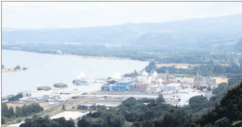
Wauna Mill as seen from Bradley State Scenic Viewpoint, just west of Westport.
