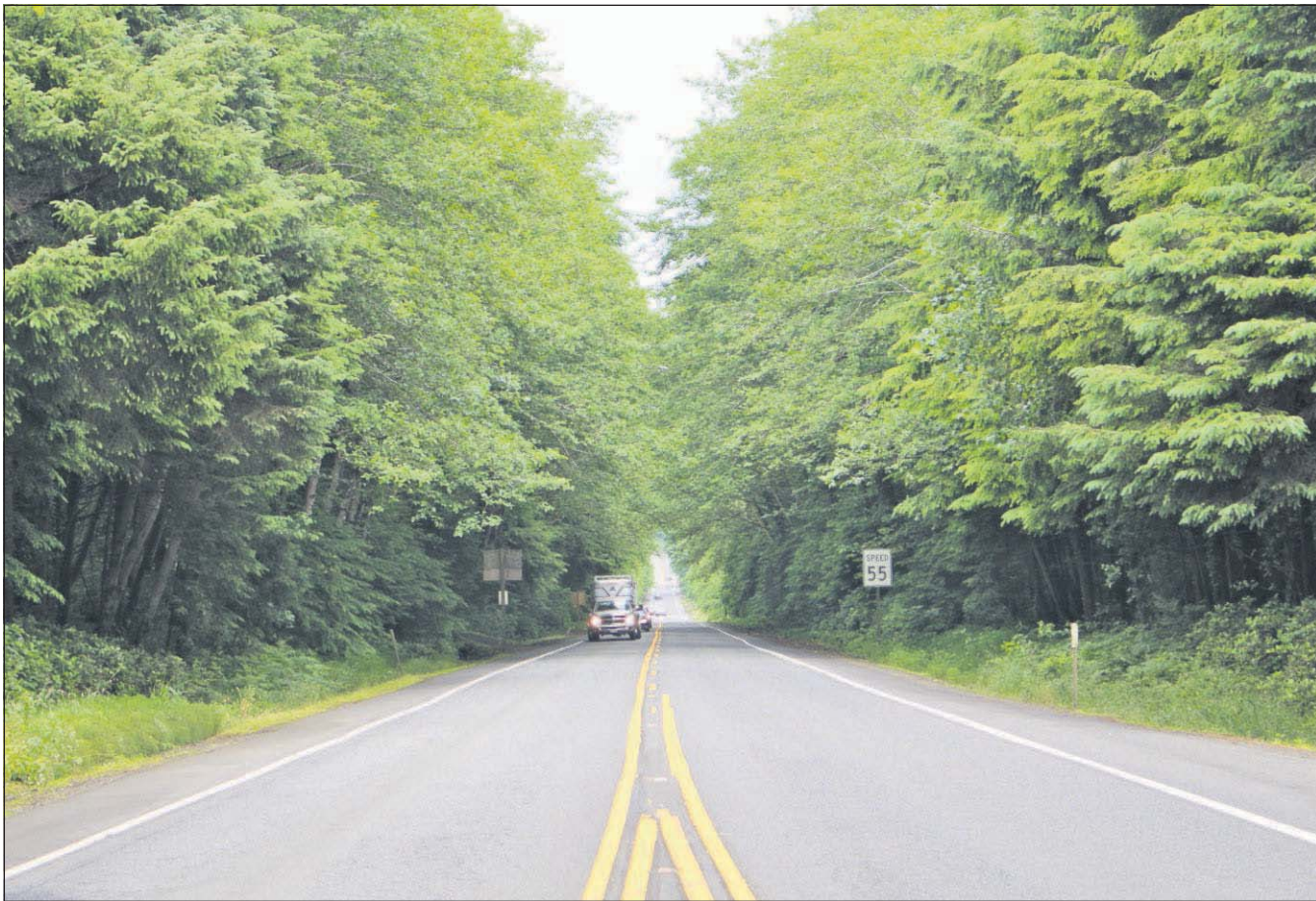
About a mile-long corridor along U.S. Highway 101 between Cannon Beach’s north entrance and Sunset Boulevard may be thinned out by the Oregon Department of Transportation. Highway officials plan to remove 200 dead and dying trees. An estimated 5,000 trees line the corridor.
