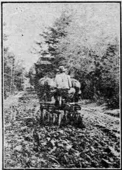
MIXING SAND AND GRAVEL.
