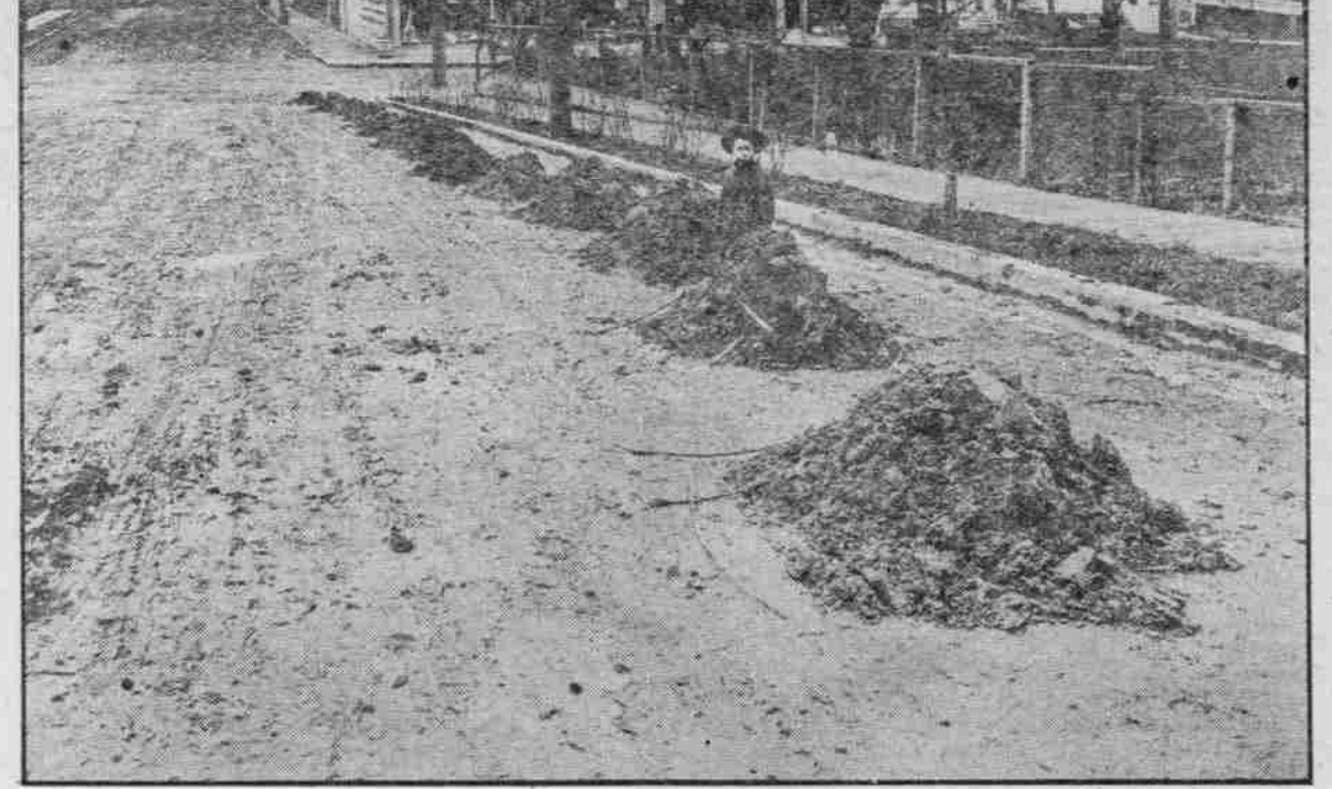
This picture presents conclusive proof that thoroughfares of city should be hardsurfaced.
