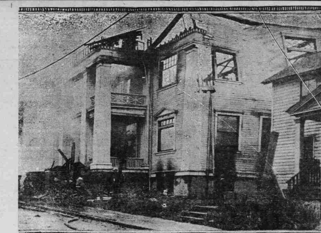
Exterior view of the building after the fire December 2. Only the four walls of the structure still stand, but the interior was completely gutted. The outside does not show heavy signs of the fire because the blaze was completely confined to the one structure.—Courtesy Oregon Journal—Photo by Ralph J. Eddy.
