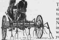
Reversing axle stubs, when reversed is like new. Reversing wheel ratchets. Removable and renewable wheel boxes. Best quality spring steel teeth. Sure self-working dump. Come and study the sturdy construction of the Champion Rake.
