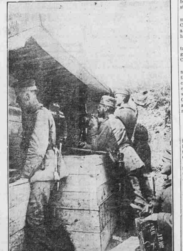
TEUTON MACHINE GUN IN ACTION UNDER BOMB-PROOF SHELTER. German gun crew operating machine gun from bomb-proof shelter of earth, grass and timber. The gun fires 400 bullets a minute and is raking the enemy's rifle pits, two hundred metres away. The gun is mounted on an elevation made of planks and filled with earth and is covered with a bomb-proof roof.
