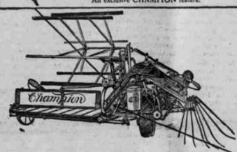
Positive Force Feed Elevator insures a positive and ious flow of grain to the packer arms. Eliminates bunching at the Binding Attachment by forcing the grain clear into the attachment. Works accurately on all weights of grain and under This is an exclusive CHAMPION feature.
