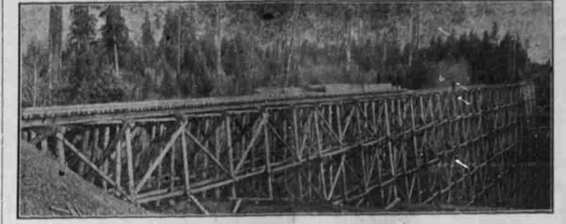
This trestle, located about a mile out of Oregon City on the new electric line is probably the largest trestle in this part of the valley. It is 123 feet high and 792 feet long. It was built early in the history of the road.
