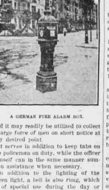
A GERMAN FIRE ALARM BOX.
