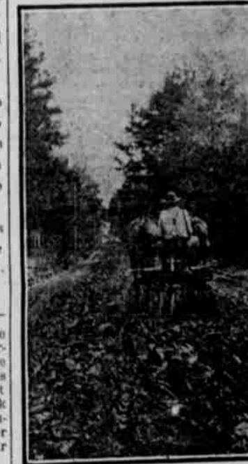
BUILDING A DIRT ROAD.
