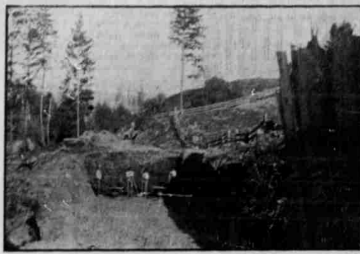
MAKING CUT ON RIGHT OF WAY TO SECURE MINIMUM GRADE
