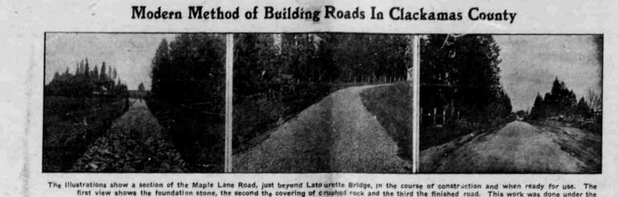
first view shows the foundation stone, the second the covering of crushed rock and the third the finished road. This work was done under the supervision of Frank Jaggar, County Road Master. The Maple Lane Road is only nine feet wide, but others recently built in the county are wider. Sections of the Oak Grove and Highland roads are twelve feet and a section of the Molalla road is sixteen feet.
