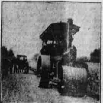
USING ROLLER ON COAL TAR ROAD.
