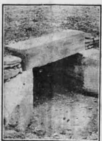
A CONCRETE CULVERT.
