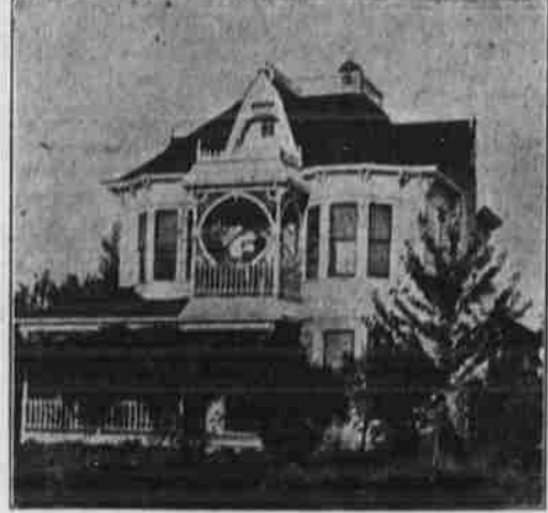
Residence of H. L. Bents.
