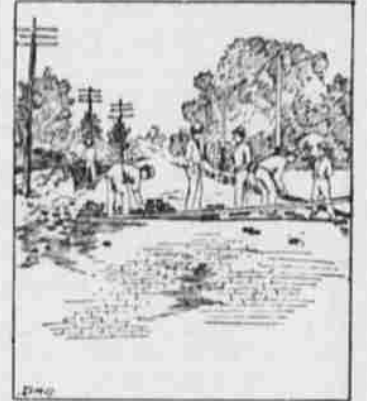
LAYING BRICK ON A SIXTEEN FOOT ROAD.
