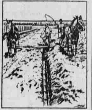
FIG. IX.—COVERING THE TILE DITCH.
