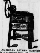
It is a departure from other rotary mo-tions. The gear is the strongest lever-age known, therefore the operation of the same is the easiest. Strain of cast-ings not known in this gear, hence breakage is eliminated. Has locking hinge gear, which locks the machine when open or closed
