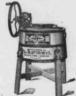
AMERICAN ROTARY WASHER. It is a departure from other rotary mo-tions. The gear is the strongest lever-age known, therefore the operation of the same is the casiest. Strain of cast-ings not known in this gear, hence breakage is eliminated. Jias locking hinge gear, which locks the machine when open or closed.
