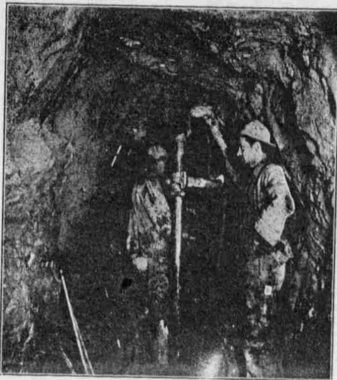
Operating Pneumatic Drill in Tunnel
