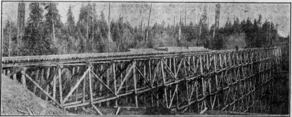
The Construction Train of the Clackamas Southern Now Passes Over the Newell Creek Canyon on One of the Finest and Most Substantial Railroad Bridges in the State. This Bridge is 792 Feet Long and 123 Feet high
