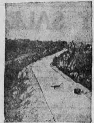
SECTION OF COMPLETED CONCRETE ROAD AT VINTON, IA.
