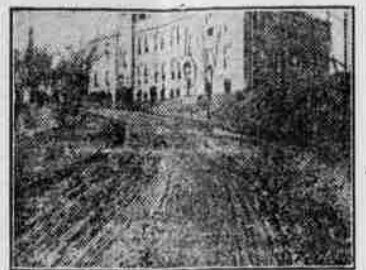
CONDITION OF A ROADWAY BEFORE USING DRAG. (From Southern Good Roads Magazine.)
