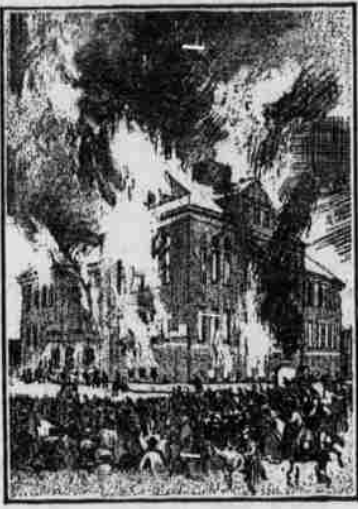
BURNING OF LAKEVIEW SCHOOL AT COLLINWOOD, O.
